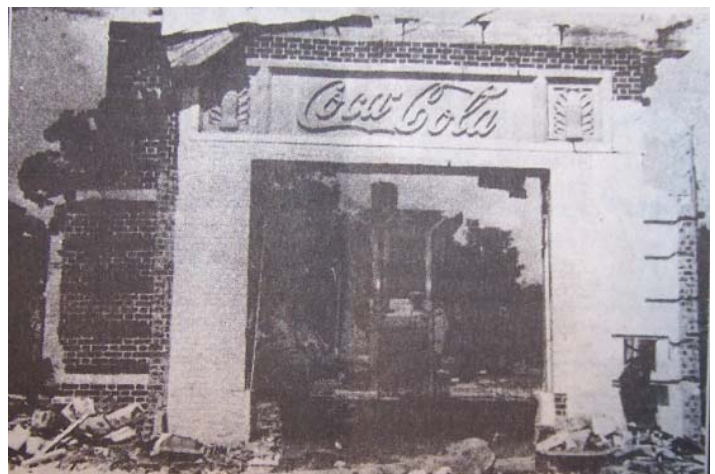
The Coca-Cola plant being demolished in 1992.
